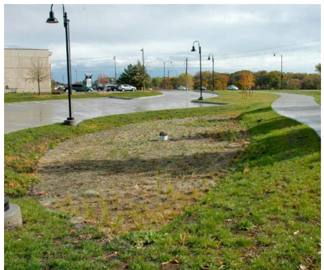
STEP 4 Planting and Mulching (Notice how deep water will pond before it overflows into the stand pipe.)
