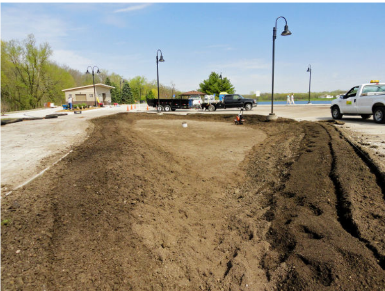
STEP 3 Placing the Soil Media
