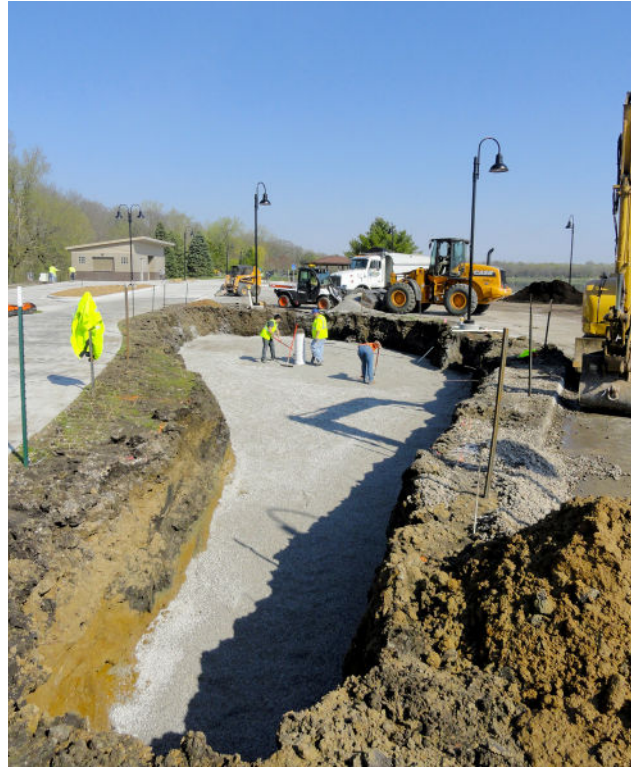
STEP 2 Installation of Rock Chamber and Overflow Stand Pipe
