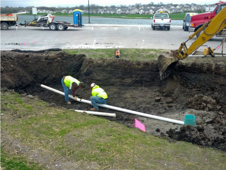
STEP 1 Excavation and Installation of the Subdrain
